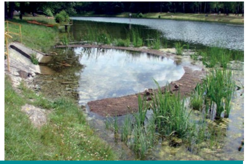
Figure 15. Buffer zone with biogeochemical barrier for the pre-treatment of water conveyed directly to the reservoir: schematic representation and pilot project in the ponds of Arturowek in Lodz
