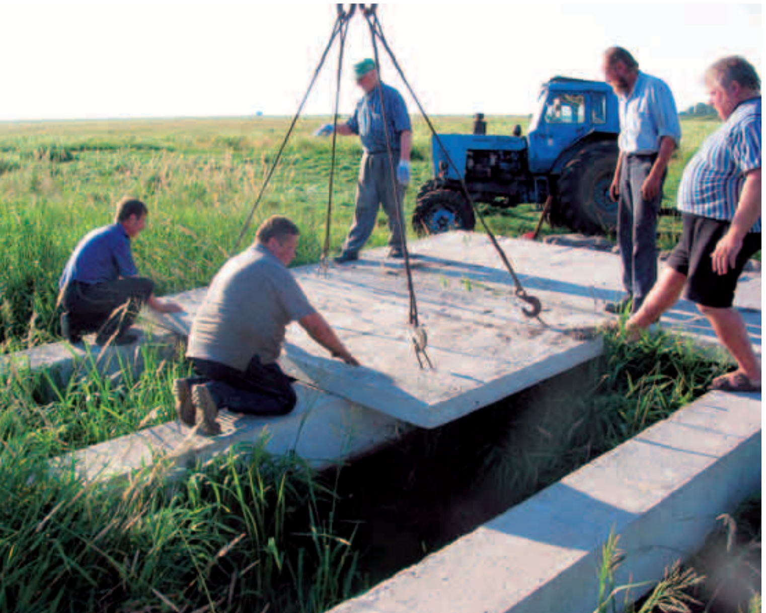
Picture IMG-0636. The biggest and principal bridge built with the help of the LIFE- project. The bridge connects parts of the coastal meadow. It has to be wide enough to let through a cattle of 100 animals and strong enough to allow a tractor with a mower to cross it.
